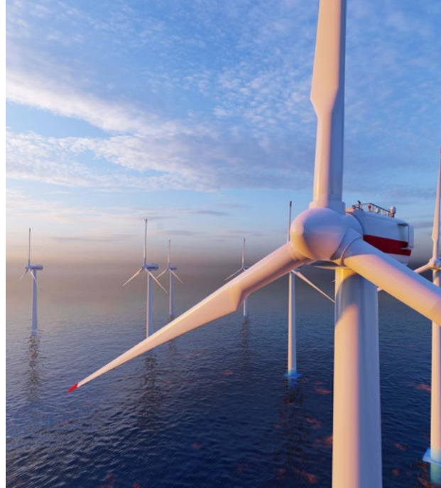
Power Management & Energy
